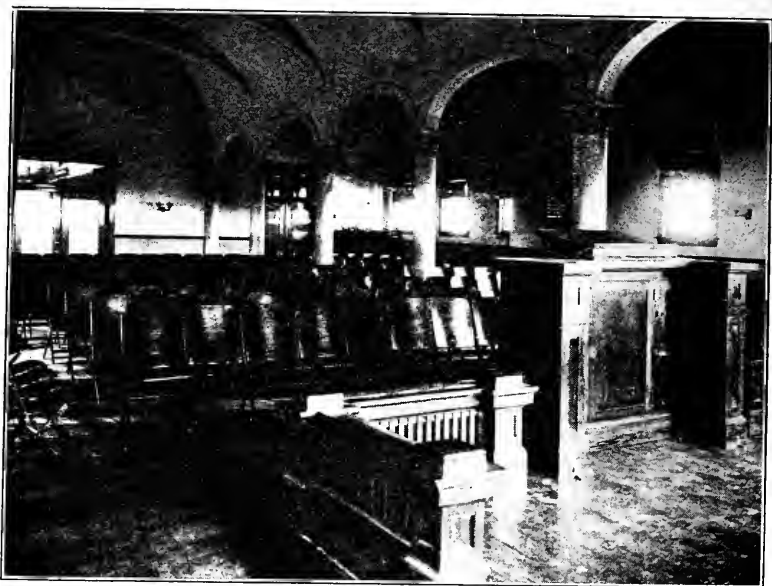
GENERAL ASSEMBLY ROOM, FOURTH FLOOR BISHOP'S BUILDING
